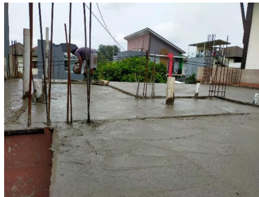
(a) Incomplete work area prior to the transition
