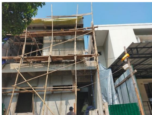
(a) Continued Building Works Under Direct Main-Contractor Execution
