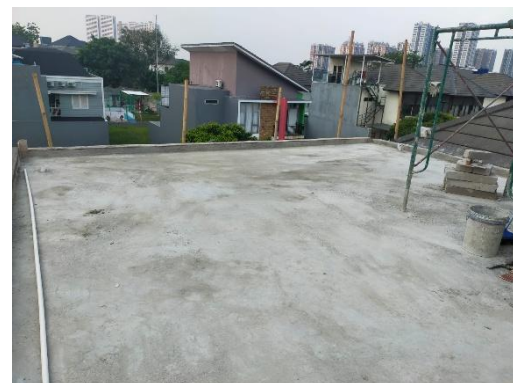
(b) Upper-Level Work Area Under Direct Main-Contractor Execution
