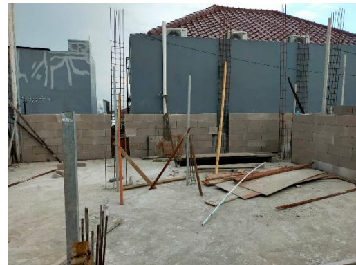
(b) Partially completed structural works prior to the transition
